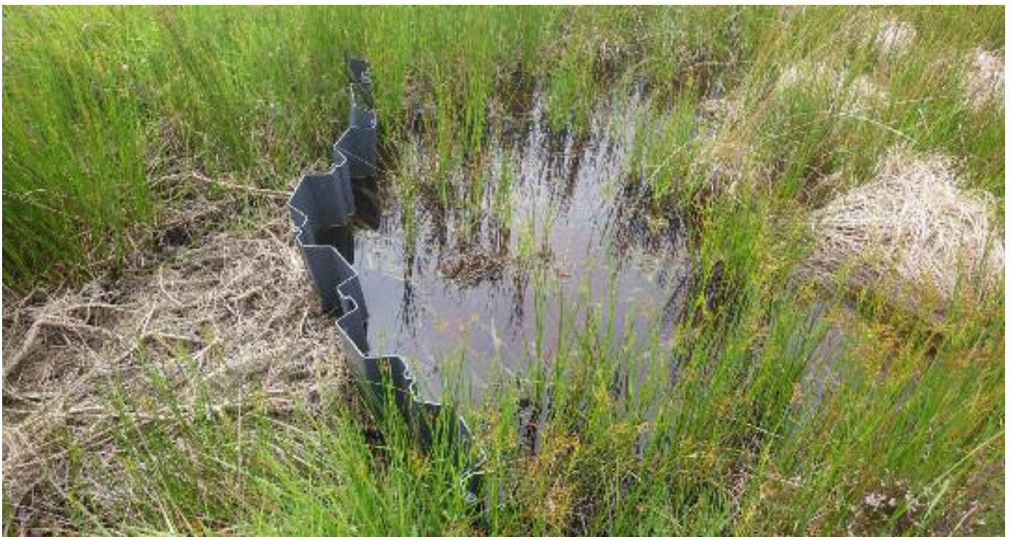
Figure 16: Photo taken in July 2017 showing water being held back by dam inserted in drain A in May 2016. Photo: K. Geraghty
