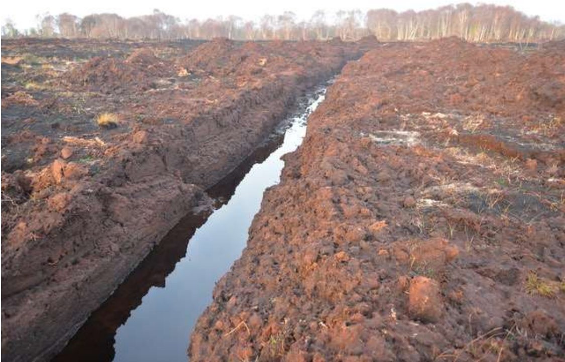
Figure 2: Peatland drainage for horticultural peat extraction at Doolistown Bog in Co. Meath 2019 without planning permission: Photo: IPCC Supporter
