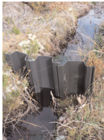
Figure 23: Drain with high water table after blocking with plastic sheet piling on Lodge Bog, Co. Kildare in 2010.
