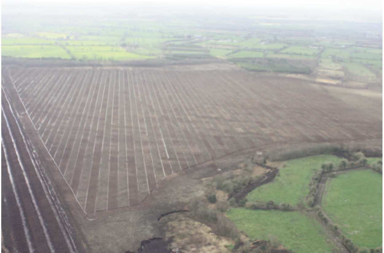
Figure 2: Air photograph looking south showing the extent of the drainage works undertaken on Clonroosk Little Bog, Cos Kildare and Offaly some time between October 2013 and March 2014.
